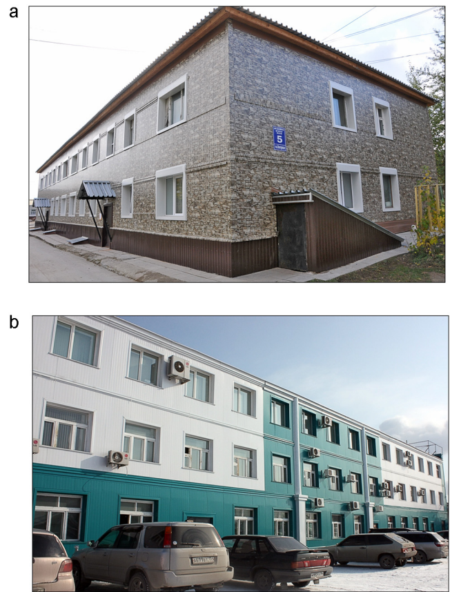
Fig. 16. A building thermally insulated with the ventilated panels: (a) a dwelling house, (b) an office block.
